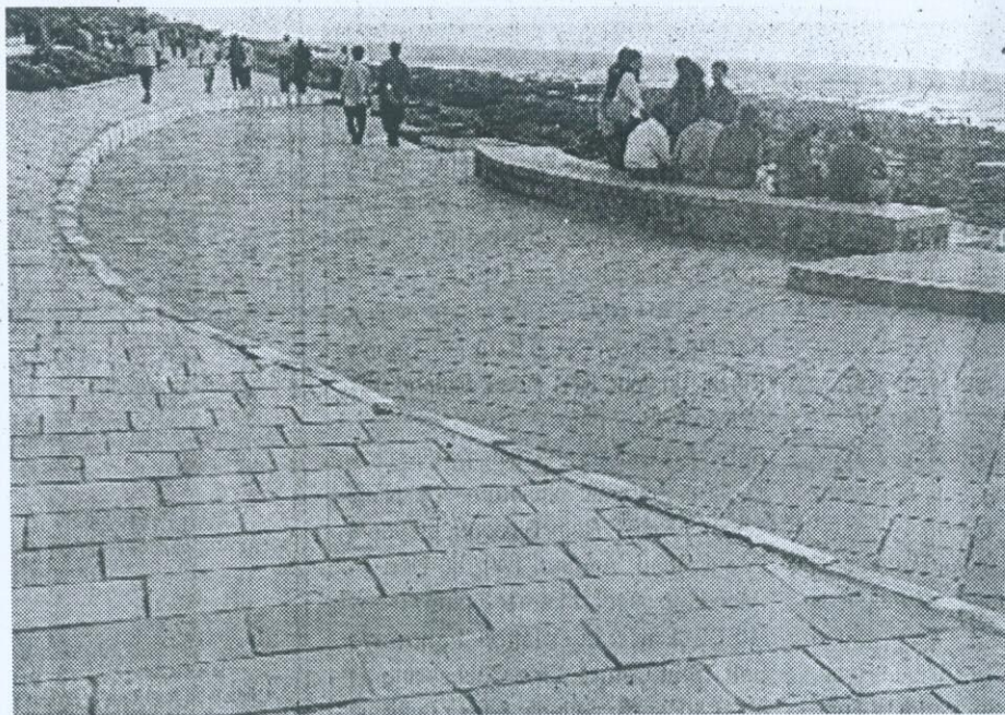
Bandra Bandstand after the redevelopment work
